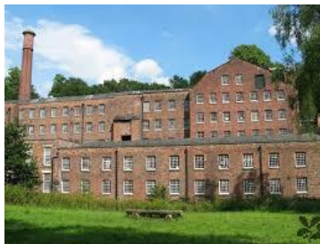
Quarry Bank Mill
